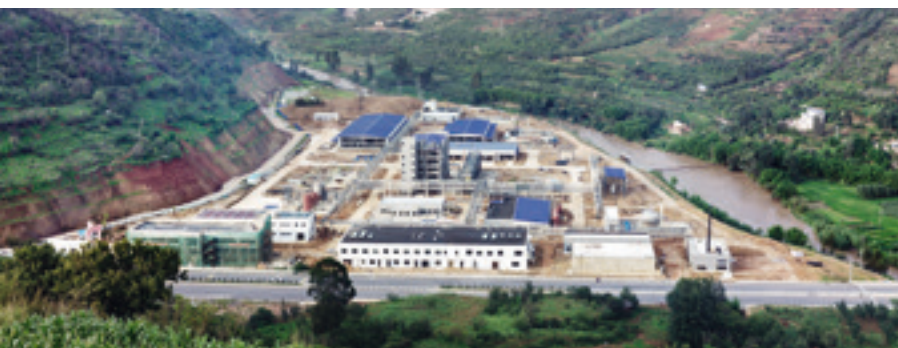
New ingredients plant in Kunming, China, (to be completed in FY15)
