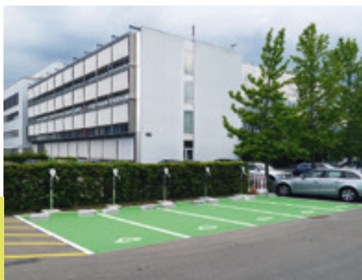
Electric car charging station at one of our Geneva sites (2014)
